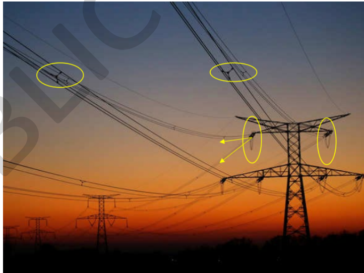
Figure 43: Clamps placements.
